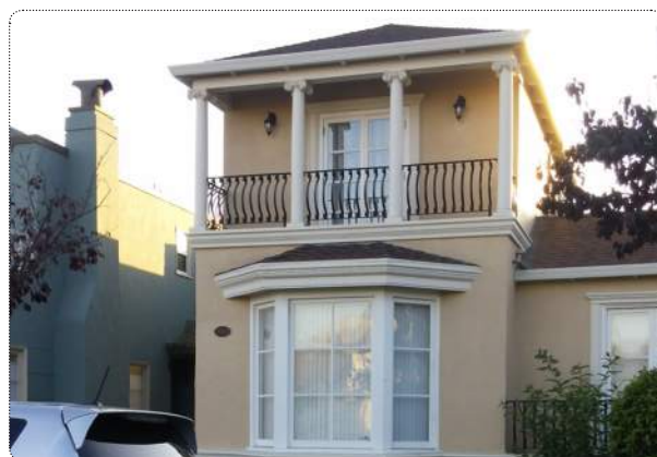
Second-story addition also added four new classical columns at the balcony, which are stylistically inconsistent.
