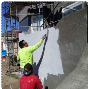
Hand-troweled stucco, as opposed to sprayed stucco, results in a higher quality finish.
