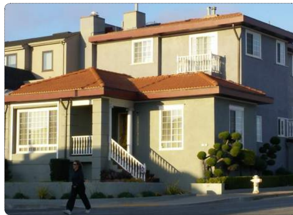
The original character of this house has been lost due to altered rooflines as well as an unsympathetically expanded building form, inappropriate replacement windows, and incompatible materials.
