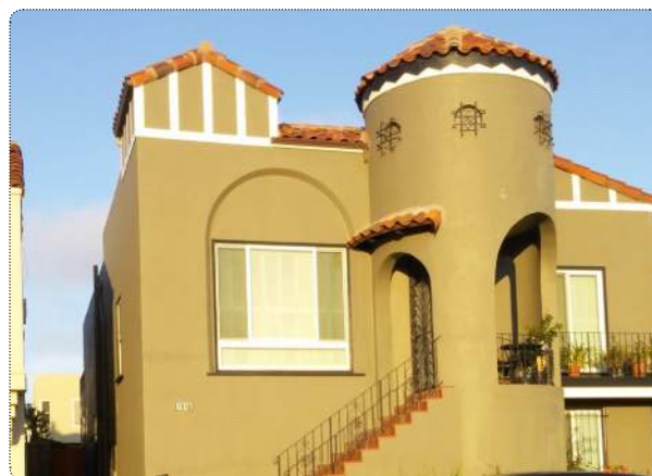
Replacement windows that are not compatible with the original wood windows detract from a building's appearance.
