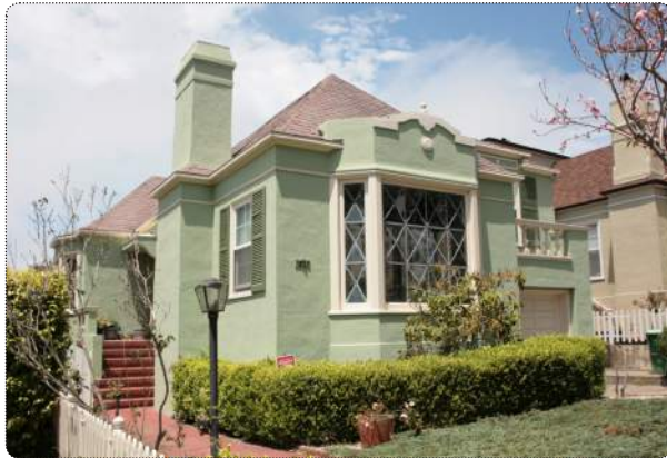
Original massing. Note that simple detail such as chimney molding and depth of eave that add richness through shadow.
