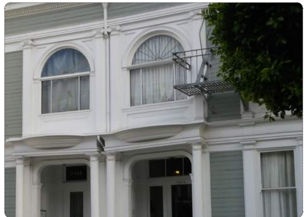
Replacement windows that do not match the glazing pattern of the original are discouraged.
