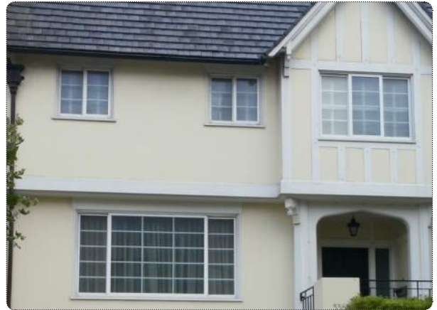
Replacement windows with simulated muntins are highly discouraged.
